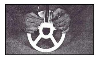
3. Insert the mounting screw through the holes in the mounting ears and pole tip—entering from the side opposite the cable connection.
